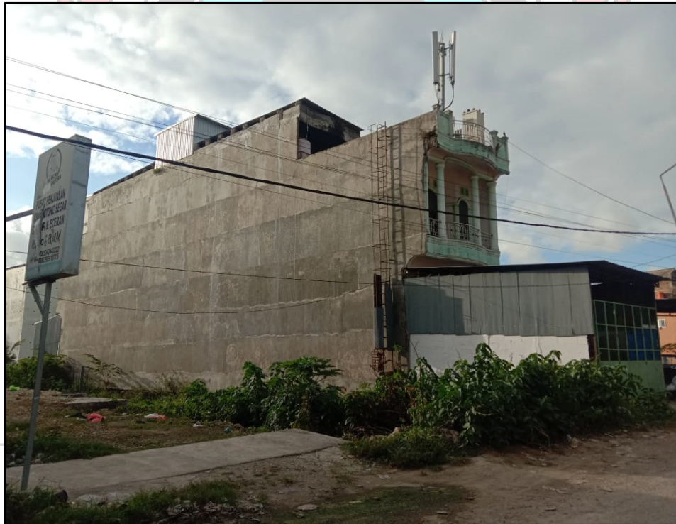
Gambar 2.1 Lokasi tower BTS rooftop Pasar Palakka Kab. Bone
