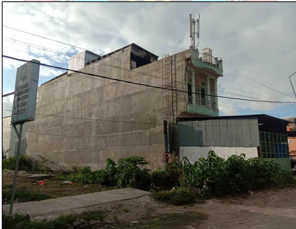
Gambar 4.1 Lokasi tower BTS rooftop Pasar Palakka Kab. Bone
