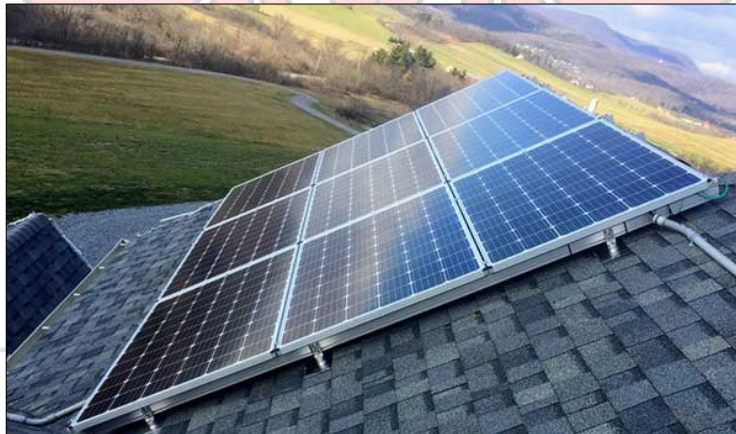
Gambar 2.14 Model pemasangan Rooftop Rack (Sumber: Builder Future Construction . 2023)
