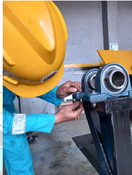
Pemasangan Bearing Pillow
