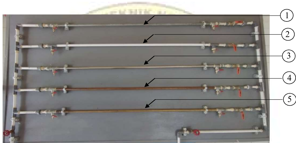
Gambar 4.1 Instalasi pipa alat uji head losses
