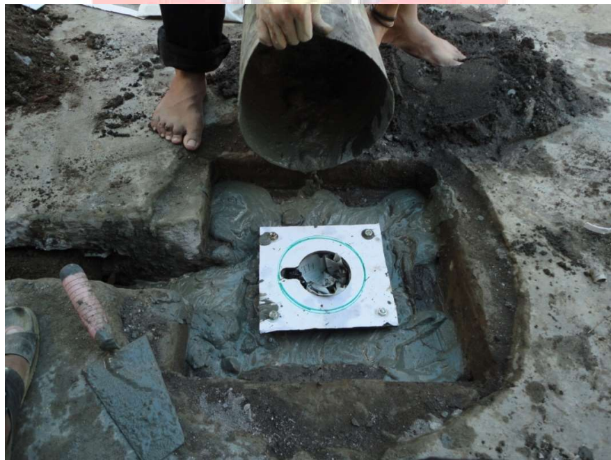
Gambar 8. Pengecoran Pitcher
