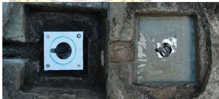
Gambar 9. Pemasangan pitcher
