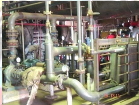
Gambar 2.10 Piping system Jacket water
