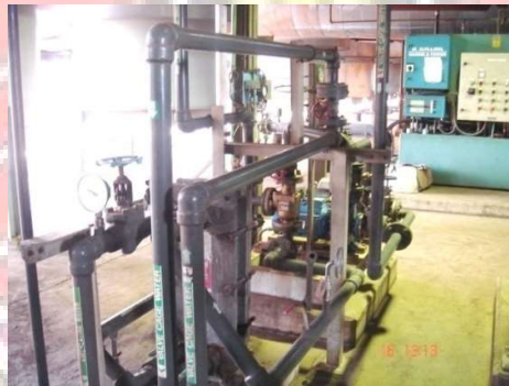
Gambar 2.12 Piping Sistem Valve Cage Water
