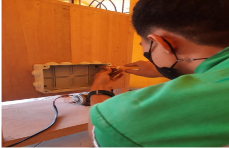
Pemasangan Box Junction
