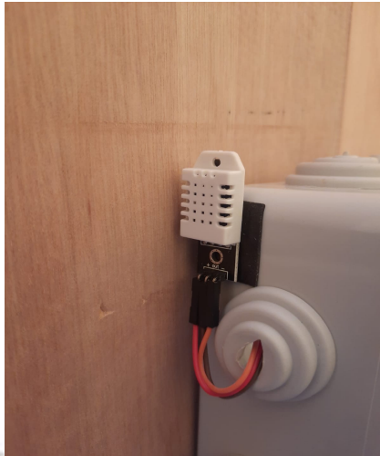
Gambar 4.7 Pengujian Sensor DHT22 di Box Dryer
