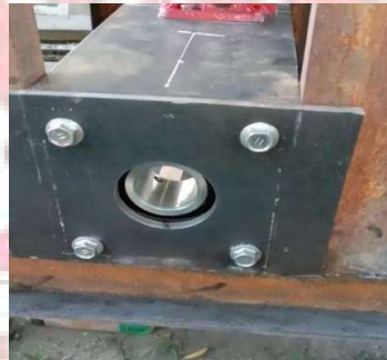
Gambar 3.2. Pemasangan Pillow Block UCF 208
