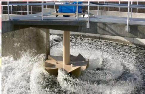
Gambar 2.3 Surface Aerator (Sumber: www.westech-inc.com )
