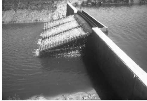
Gambar 2.4 Gravity Aerator (Sumber: www.ebrary.net )
