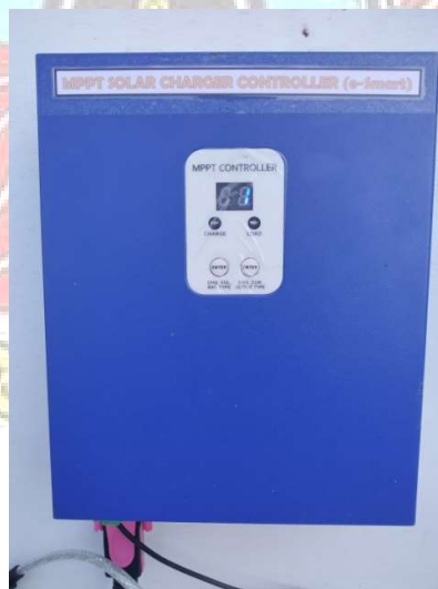
Gambar 4.11 MPPT Solar Charge Controller
