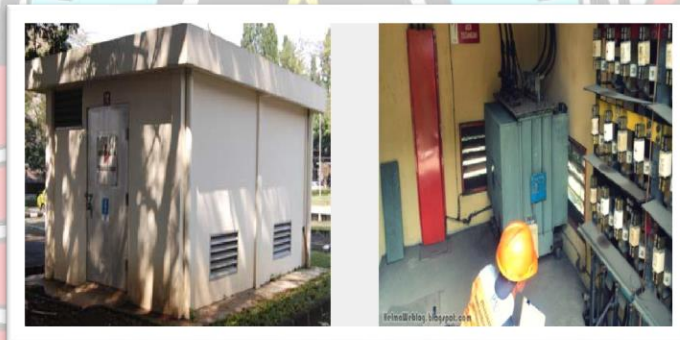
Gambar 6. Gardu beton
