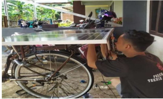
Gambar 9 Proses perakitan panel surya
