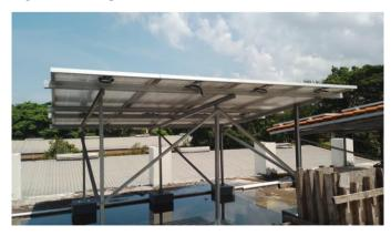
Figure 5. 3 kWp Solar Panel-1
