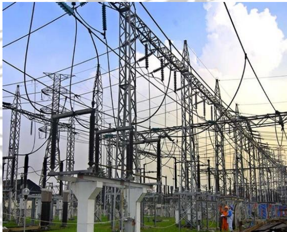
Gambar 13 Rel Daya ( Busbar )
