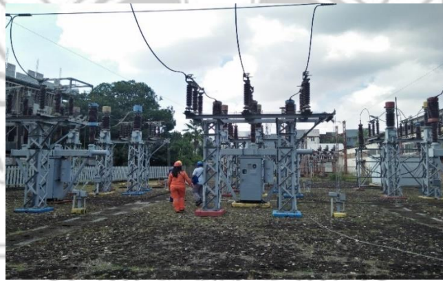
Gambar 29 Peralatan GI Konvensional 150 KV Bontoala
