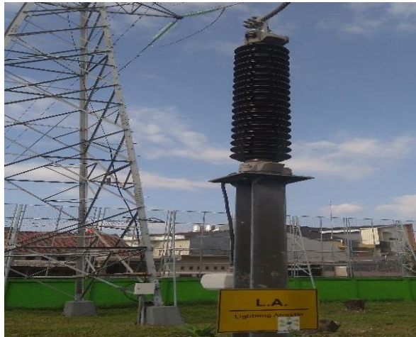
Gambar 8 Lightning Arrester (LA)
