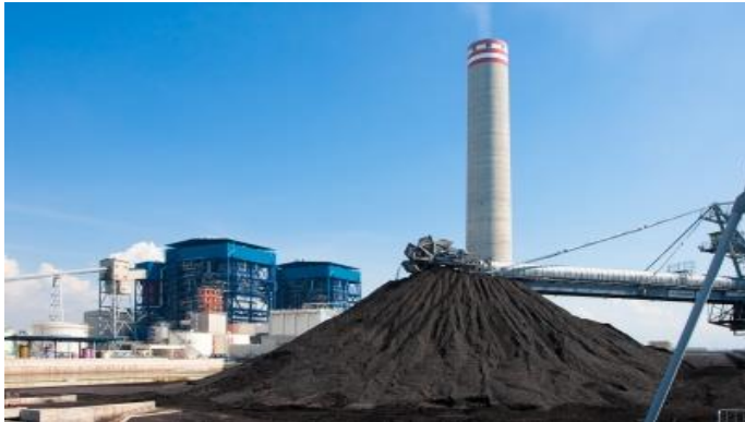
Image: Coal-fired power plants use steam coal as source to generate electricity. Photo courtesy of John Kasawa/FreeDigitalPhotos.net.
