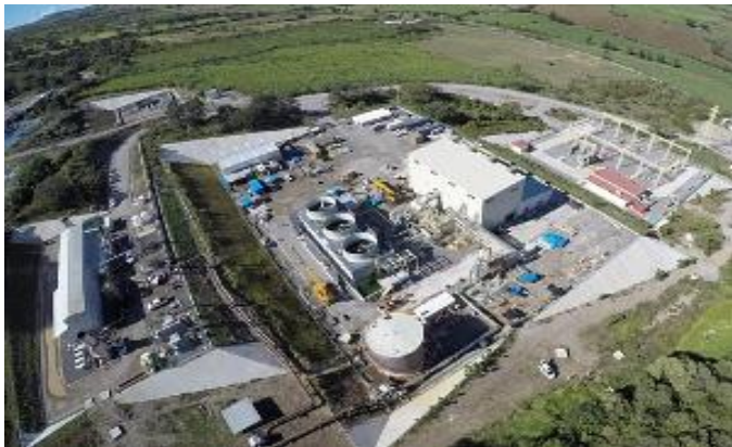
Image: The Domo de San Pedro geothermal power plant in Mexico. Photo: courtesy of Grupo Dragon/Mitsubishi Hitachi Power Systems, Ltd.
