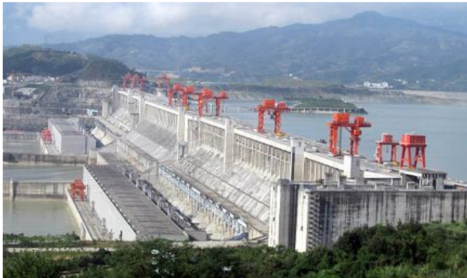
Image: The 22,500MW Three Gorges hydroelectric power plant in Yichang, Hubei province, China. Photo courtesy of http://www.power-technology.com .
