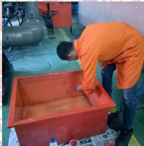
Pengecatan reservoir
