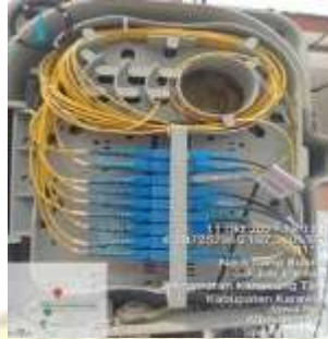
Gambar 2. 8 Optical Distribution Point (ODP)
