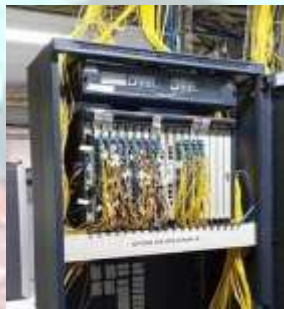
Gambar 2. 5 Optical Line Terminal (OLT)
