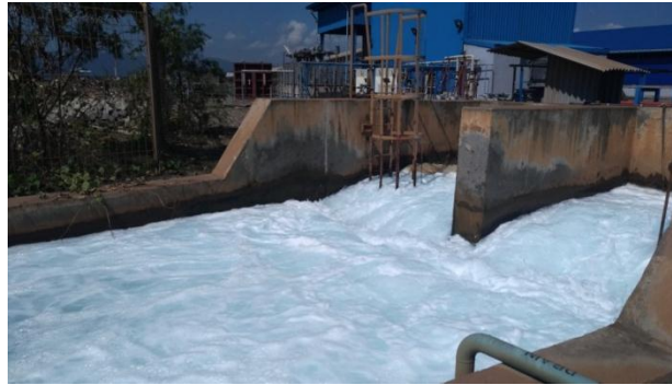
Fig. 1: Waste Water Pit (PT. Antam, 2016)
