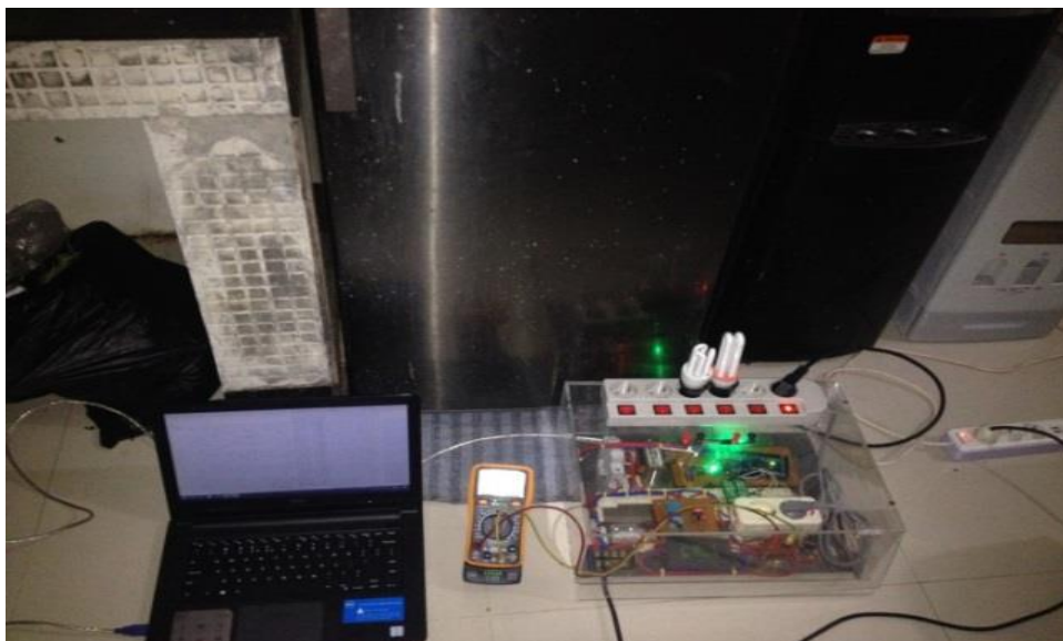
Fig 4. Testing Dispenser Loads
