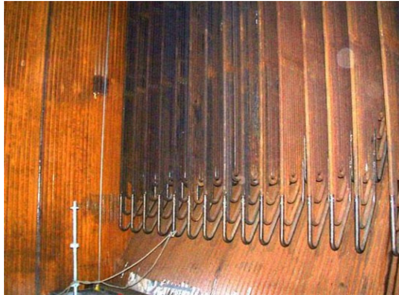
Gambar 2.13 Panel superheater . (Sumber: Teir, 2003)
