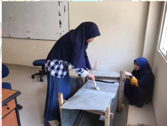
Pengecatan Rangka Ducting
