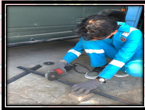
Gambar 4.5 Memotong besi
