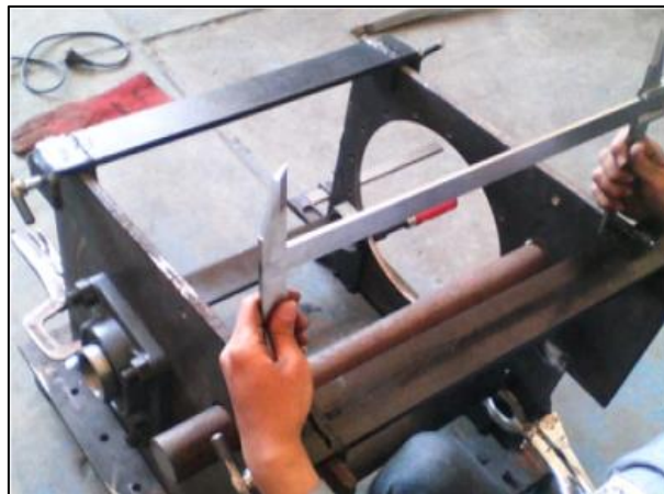
Figure 4. Measurement before welded
