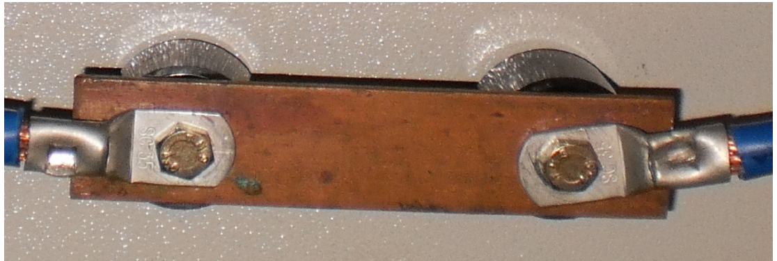
Gambar 19. PEB (Potential Equalizing Bar)
