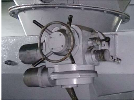
Gambar 2.14 Motor Operated Valve (MOV) . Sumber : PLTU Barru.
