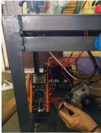
Test Negative Side of Charging Circuit
