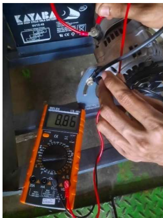
Check System Voltage
