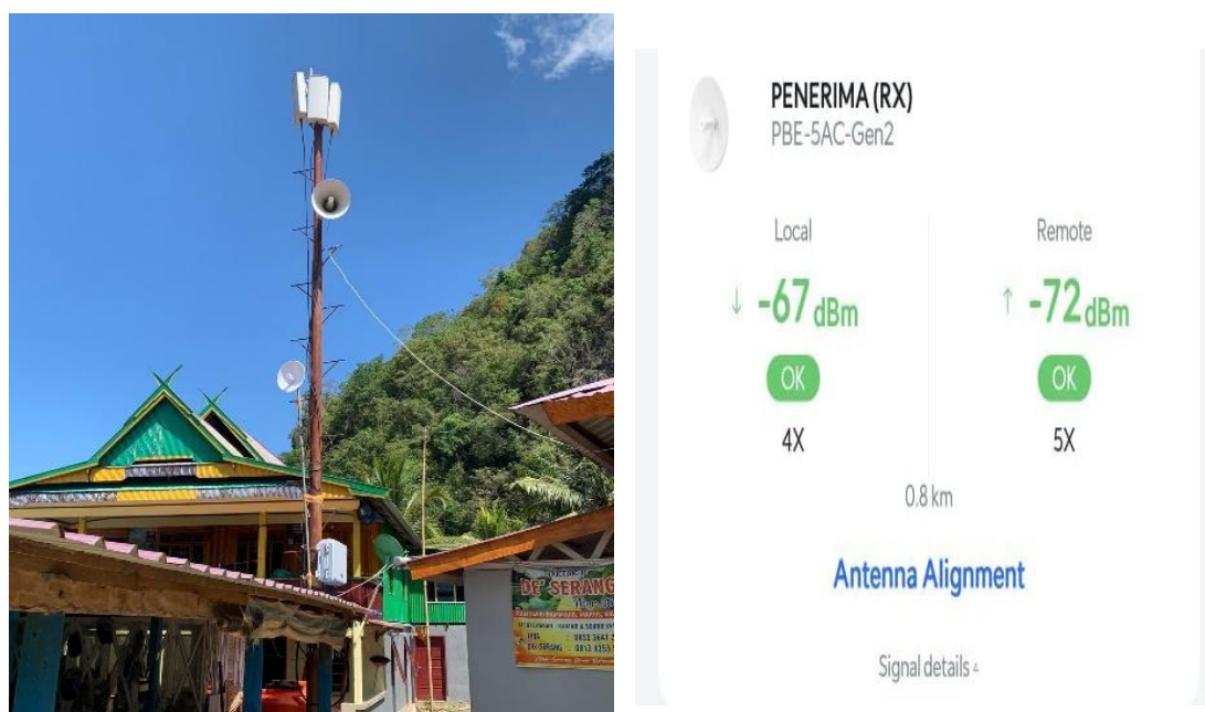
FIGURE 6. RM-Rx and its antenna configuration
