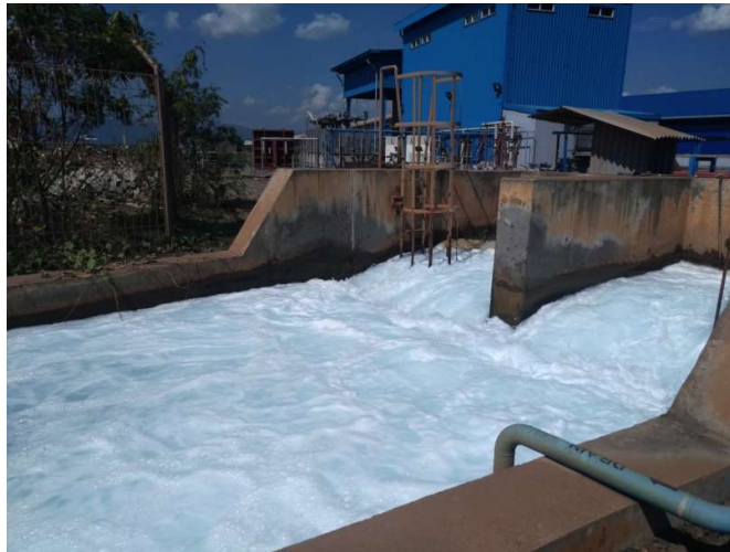
Gambar 2.3 Waste water pit PLTU ANTAM Tbk.
