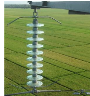
Gambar 3. Arcing Horn
