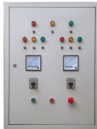
Gambar 5. Tampak depan panel ATS/AMF
